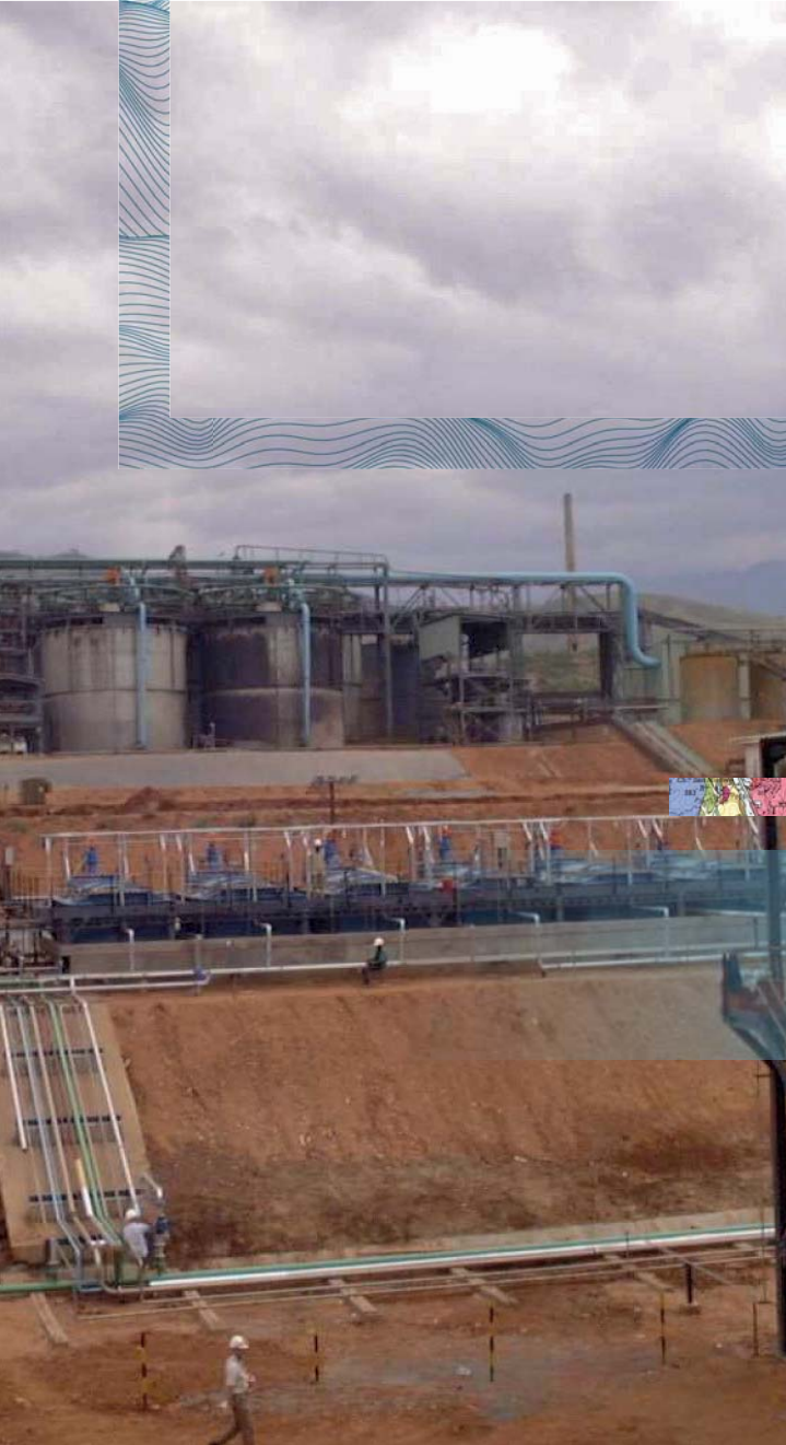
Bioleaching for the recovery of cobalt from cobalt-bearing pyrite (KCC Project, Uganda). © BRGM – Dominique Morin
