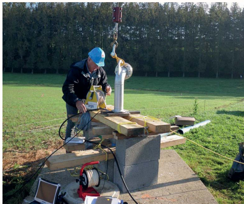
Borehole equipped with measurement systems (Brittany, 2011). © BRGM - Bruno Mougin
